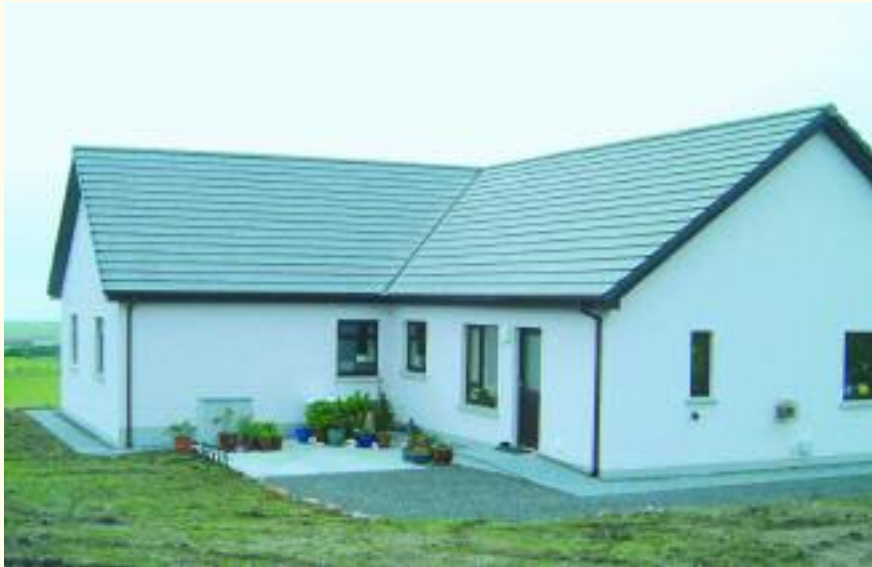
Completed WALLFORM home
