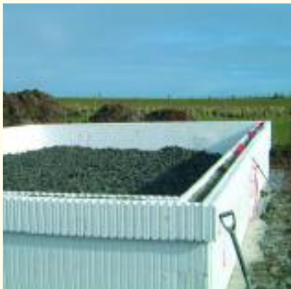
WALLFORM substructure on concrete foundations.
